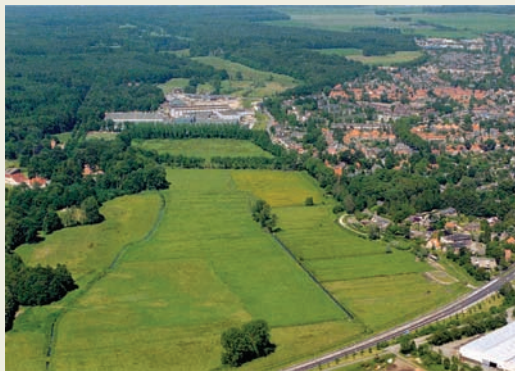
The Renkum brook valley before restoration
