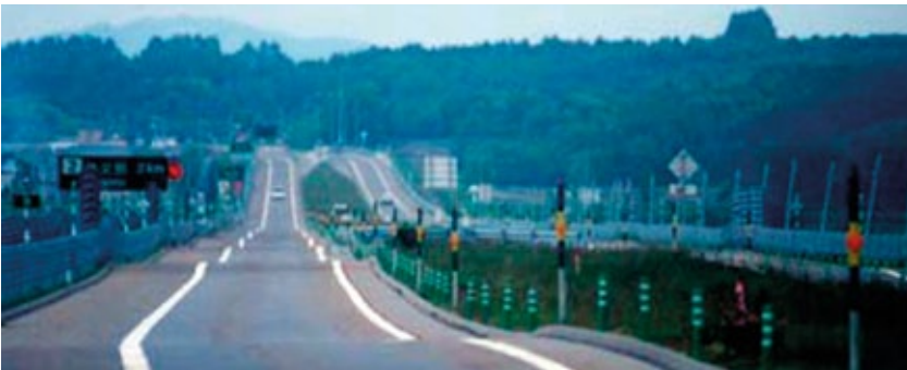
Fig. 1. Uneven subsidence of highway
