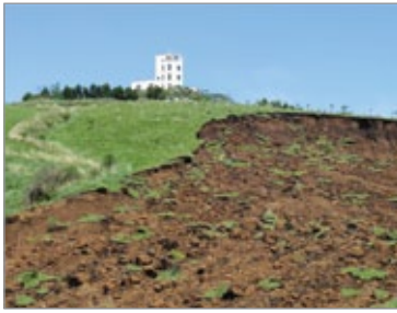
Photo1. Large landslide flows on the gentle slopes
