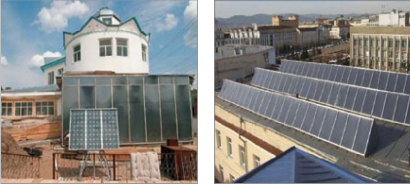
Fig. 2. Photocells and solar panels on private house (Ulan-Ude) — A. Sun collectors on the roof of the hotel “Baikal Plaza” area of 150 m 2 (Ulan-Ude) - B.
